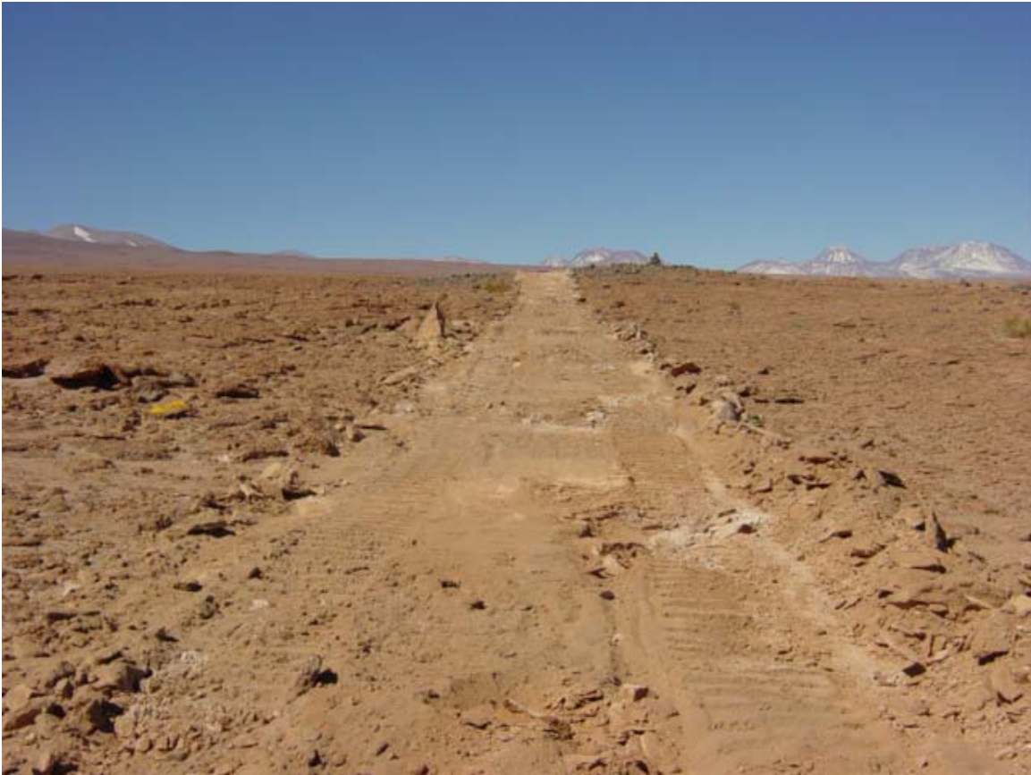
Road Opening Between the Public Road and the OSF
